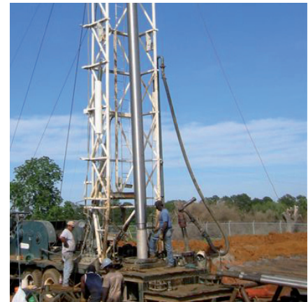
Installation of the Muni-Pak
